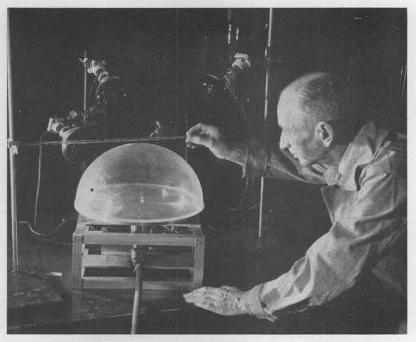
AIR AND INFRA-RED LIGHT are used to form a sheet of plastic into the half sphere shown in this picture. The plastic is held on a revolving platform as air is forced in from below. At the same time the infra-red lights heat the plastic to make it pliable.
